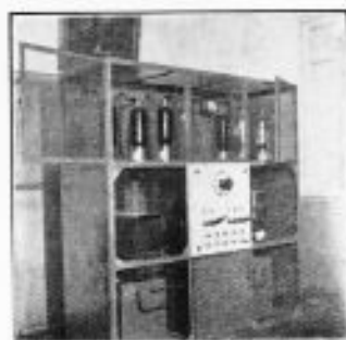
Tube rectifier at the station „Maly Komintern.”
