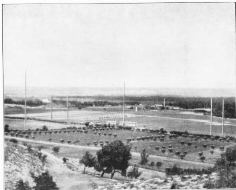
General view of the „Compania Nacional de T. S. H.” 25 kW. CW. valve transmitting station at Aranjuez (Madrid) used for the international service with England, France, Italy, Switzerland, Germany and Austria.
